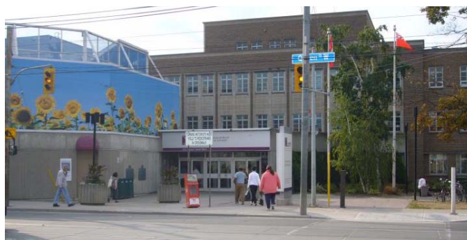
Above: CAMH's existing Administration Building, the Workman Theatre is at left.
